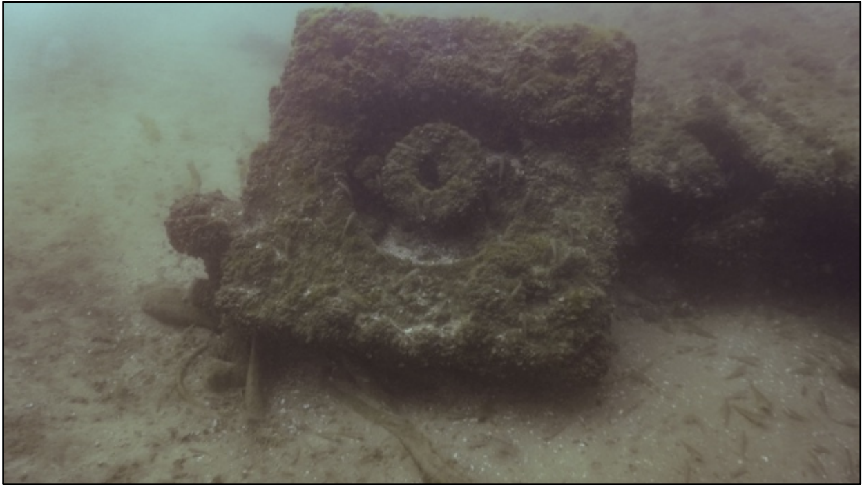
Figure 11. Invasive mussel coverage on metal features.
